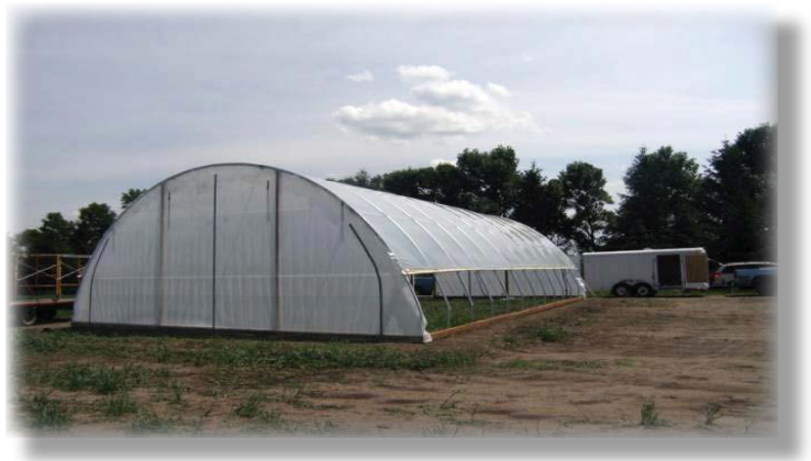
A seasonal high tunnel is a polyethylene covered structure used to create favorable growing conditions.
